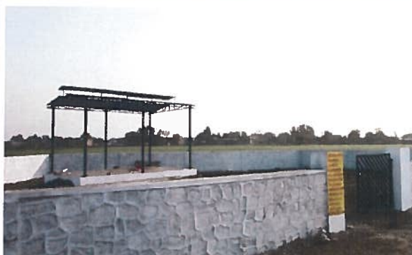
Community Toilet Block at Simliya village
